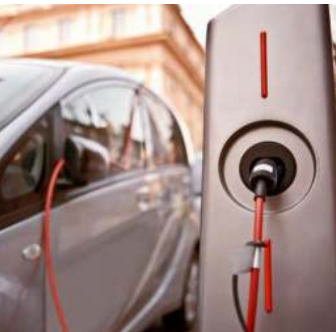
Electric car charging station.
